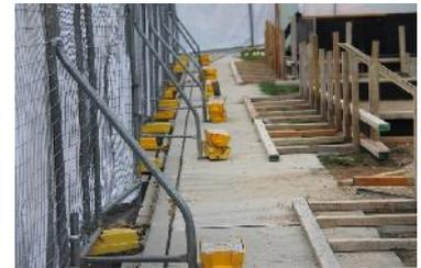
Photos show examples of braced temporary fencing with shade cloth attached
